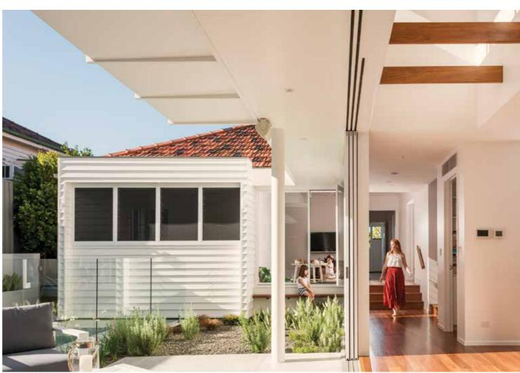
onto the building, creating a textural effect which is reminiscent of the play of light on the original weatherboards. Deep eaves to the upper level also protect against sun and rain, allowing the windows to be left open even when the heavens open.
